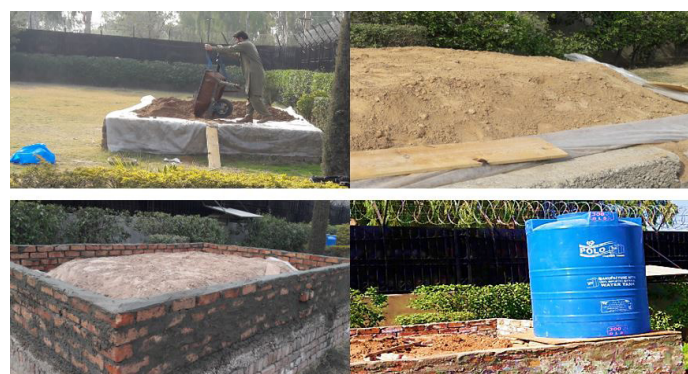
Figure 3: Lab plantation, construction of planter and soil bed preparation. Preventing seepage losses using plastic sheet. Masonry work around the perimeter to isolate the site and maintain a constant water depth during plants growth.
